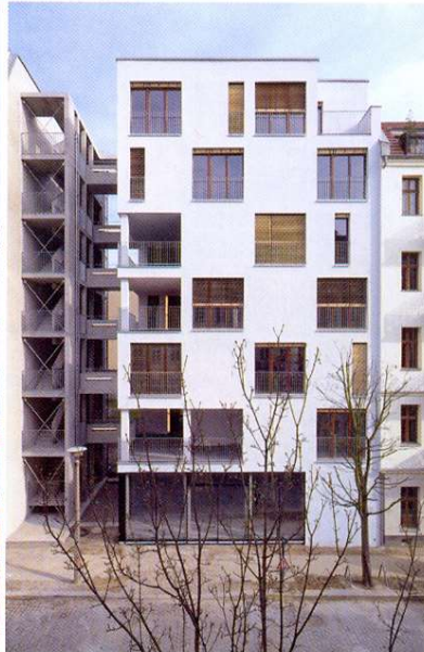
Multi-storey housing by the building cooperative e3, Berlin, 2008; architects: Kaden + Klingbeil 4th floor plan scale 1:400
