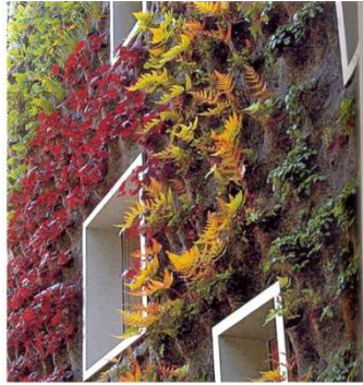
Hydroponic System with Felt Substrate on Timber Wall Construction
