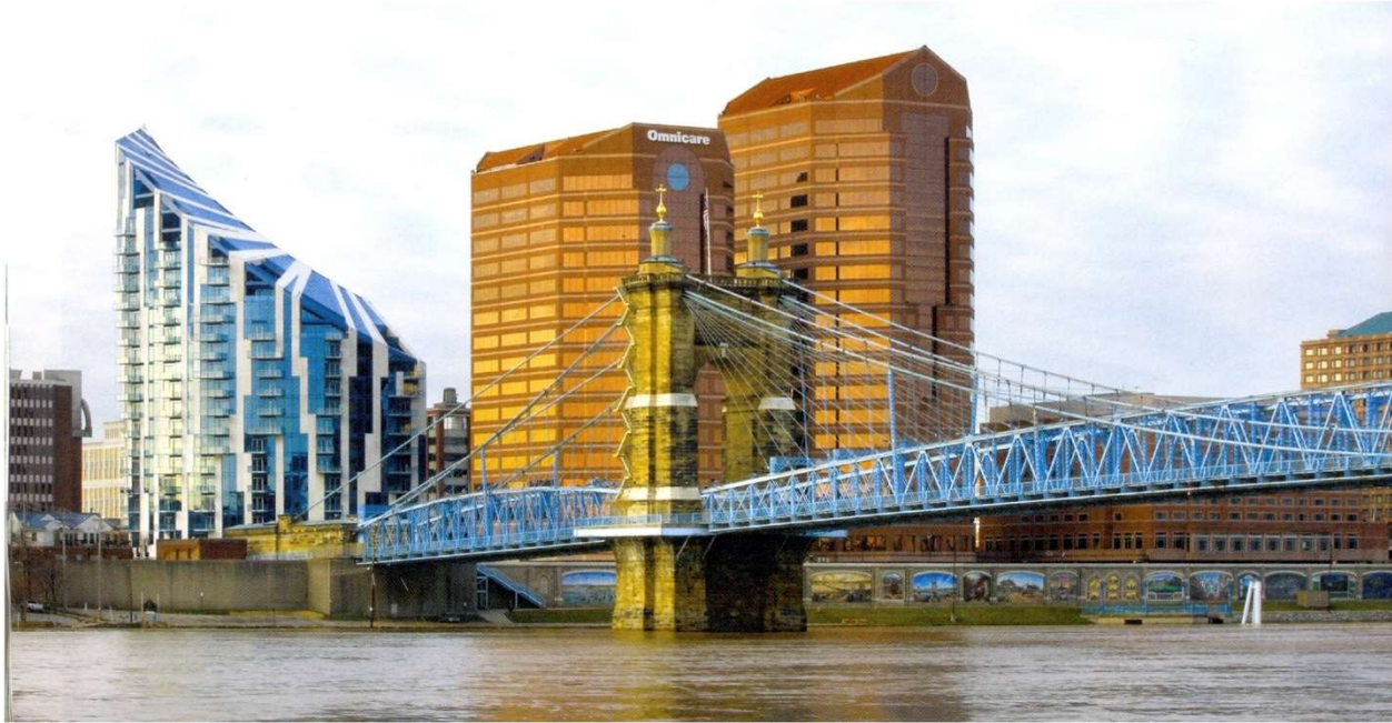
The ascent at Roeblings Bridge, Covington, Kentucky, USA 2008, Architect : GBBN Architects
