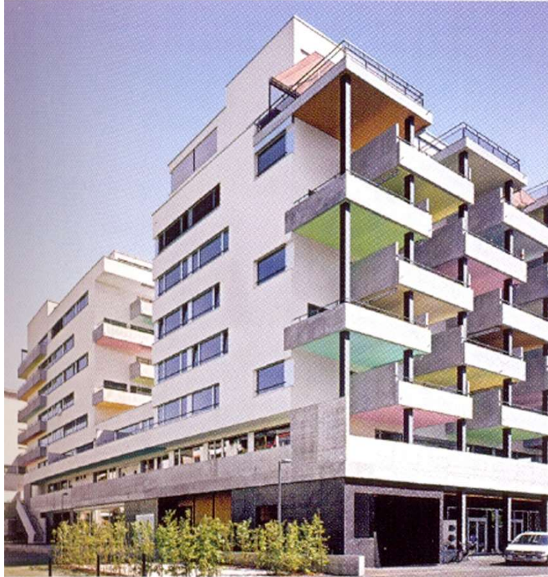
James housing development, Zurich, 2006 architects: Gmür and Geschwentner, Zurich
