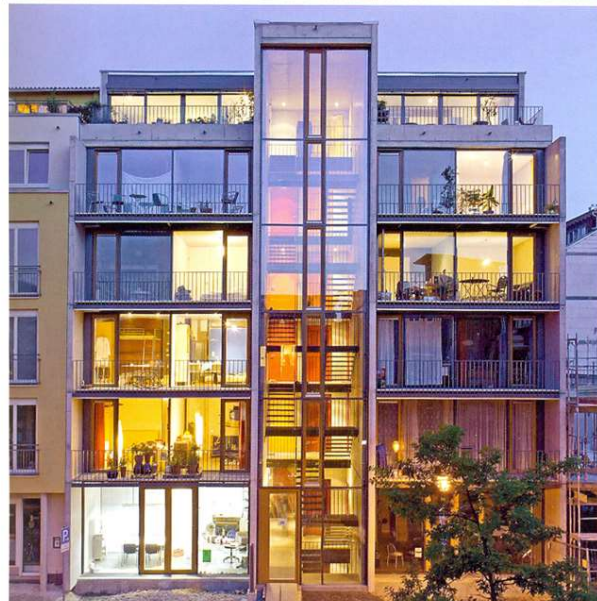
"Prisma" multi-family housing, Tübingen, 2004; architects: Noerenalbus Architecture
