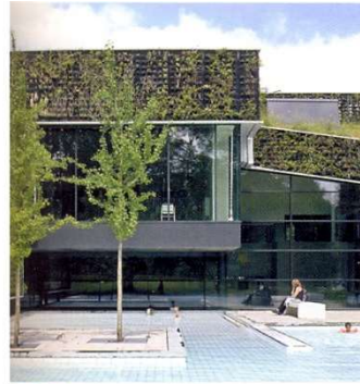
Hydroponic System with Felt Substrate on Steel Constructions
