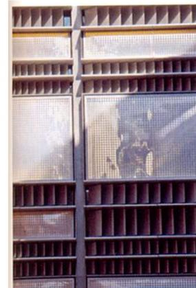
*The buildings are oriented to provide optimum shade and reduce cooling loads and shaded colonnades at podium level bring benefits through high insulation and exposed thermal mass.*
