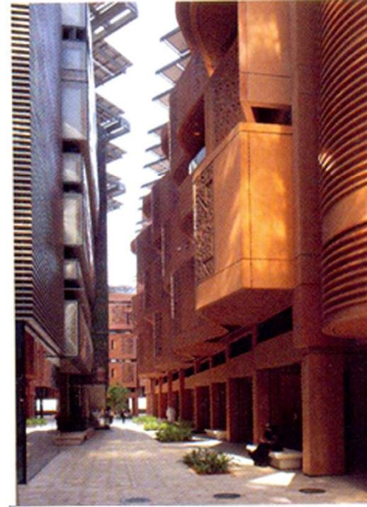
*The ratio of open facade areas and exposed upper areas. Openings in the facade vary according to their position – the upper floors are more solid, with approximately 25% glass, while the shaded lower floors have a greater proportion of glazed area, around 45%.*
