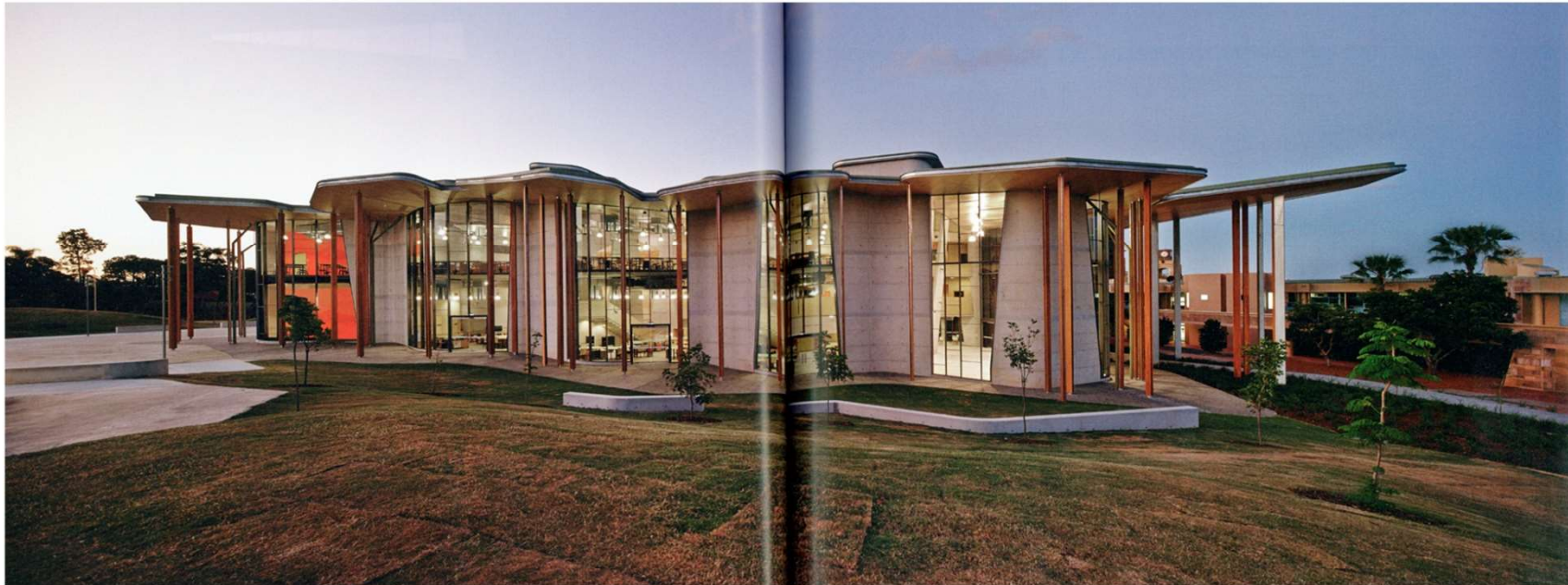
Street Scene. School of architecture, Bond University. Brisbane, Australia. Архитектурная школа. Брисбен, Австралия Architects: CRAB studio
